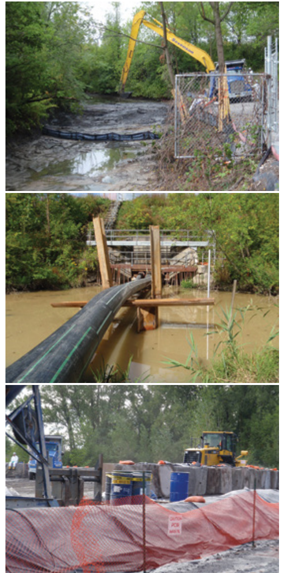
FIGURE 4.16: Top photo: Water was removed from Beaverdams Creek by channelling its flow through a large pipeline. Workers were then able to remove the contaminated sediment from the creek bed and restore the creek to more natural conditions. The planting of trees and shrubs restored vegetation in the area and the addition of logs in the creek improved fish habitat. Middle photo: The pipeline channelling water from upstream areas ensured flow remained in downstream areas of Beaverdams Creek. Bottom photo: PCB-contaminated sediment was brought to a staging area where it was dried and hardened for safe transport to a hazardous waste facility for proper disposal.
